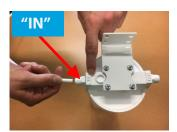
1. Using a sharp knife and the 1/4" tubing provided, cut a length of tubing to the proper length to connect the T-Valve to the elita canister. Insert one end of the tubing into the Quick Connect Fitting (QCF) on the T-Valve and the other end into the QCF labeled "IN" on the elita housing lid.
